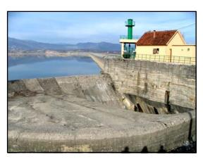
HPP Perucica is combination reservoir-derivation system, constructed near Glava Zeta. Catchment area of hydro-geological basin of Niksic field is 894 km<sup>2</sup>, while mean annual discharge of stream flow is 34.8 m<sup>3</sup>/s. Installed capacity of HPP Perucica is 307 MW, while available is 285 MW.
